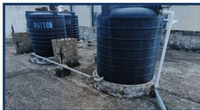
Fig. 1 : Drinking water storage tank
